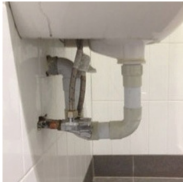
POOR PLUMBING MARK OUT
