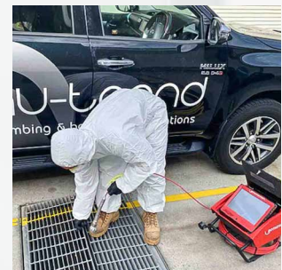
NU-TREND CAMERA INSPECTION AND JET BLAST
